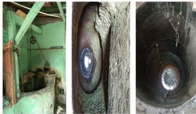
Figure 2. Dug Well with Dipper
